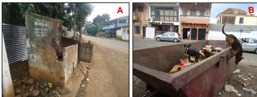
Fig. 2. Examples of inadequate collection equipment use in São Tomé island: (a) damaged fixed MSW storing compartment due to lack of maintenance; (b) an open container for street use, becomes an attracting hotspot for animals.
