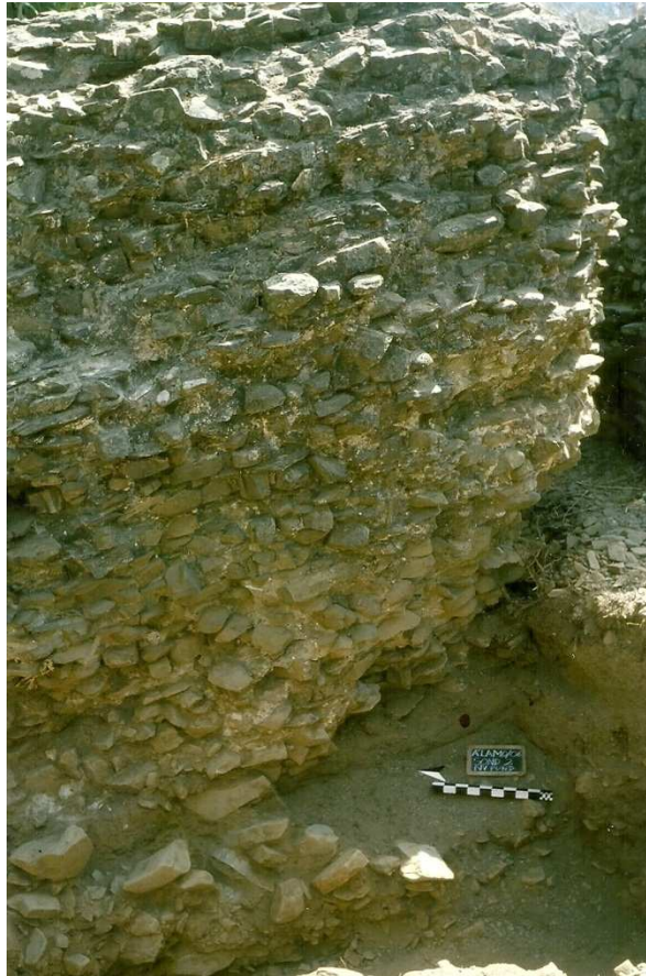
Figure 14. Dam of Álamo. Detail of Survey 2 (2006). Note the existence of fine sediments under the basement of the collapsed section of the wall by the waters of the Ribeira da Foupana that currently crosses the structure through the existent fissure. Photo J. L. Cardoso.
