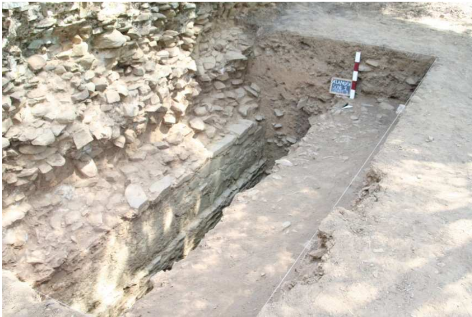
Figure 4. Partial view of Survey 1 (2006), showing the contrast between the conservation of the upper part of the upstream wall and the lower part, interred in the sediments accumulated at the bottom of the reservoir. Photo J. L. Cardoso.
