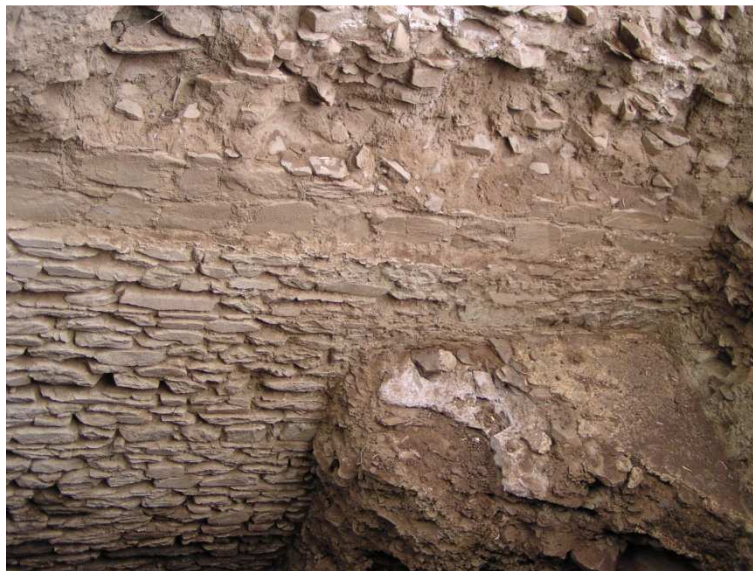
Figure 19. Dam of Álamo. Partial view of two layers of mortar, in the middle of the ancient reservoir near the upstream wall, made over the deposits accumulated at the bottom of the reservoir. See Fig. 5. Photo J. L. Cardoso.
