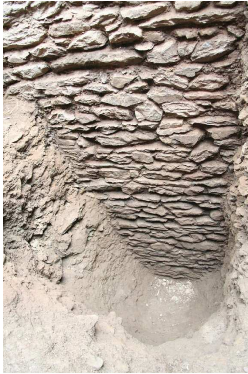
Figure 17. Dam of Álamo. Detail of the upstream wall built with isometric blocks of greywacke ( opus incertum ), observed at Survey 4 (2007). Note at the bottom the geological substratum. Photo A. Gradim.
