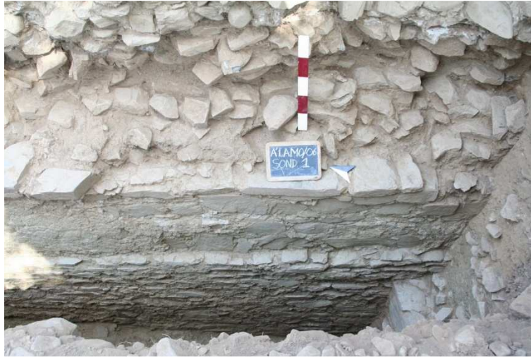
Figure 8. Dam of Álamo. Partial view of the upstream wall, observed in Survey 1 (2006), with a small longitudinal step. Photo A. Gradim.
