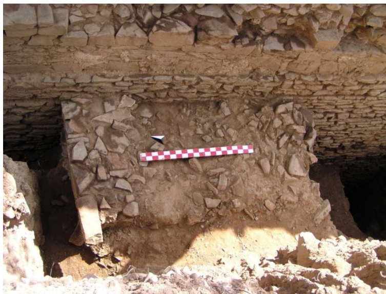
Figure 11. Dam of Álamo. View of the platform observed in the middle of the upstream wall. Photo J. L. Cardoso.
