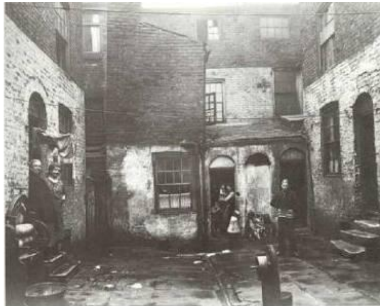
JOHNSON'S COURT, 1935. A typical tenement with no indoor sanitation and a single tap to service all the flats below. Showing some of the very insanitary legacy of the industrial revolution in Liverpool.
