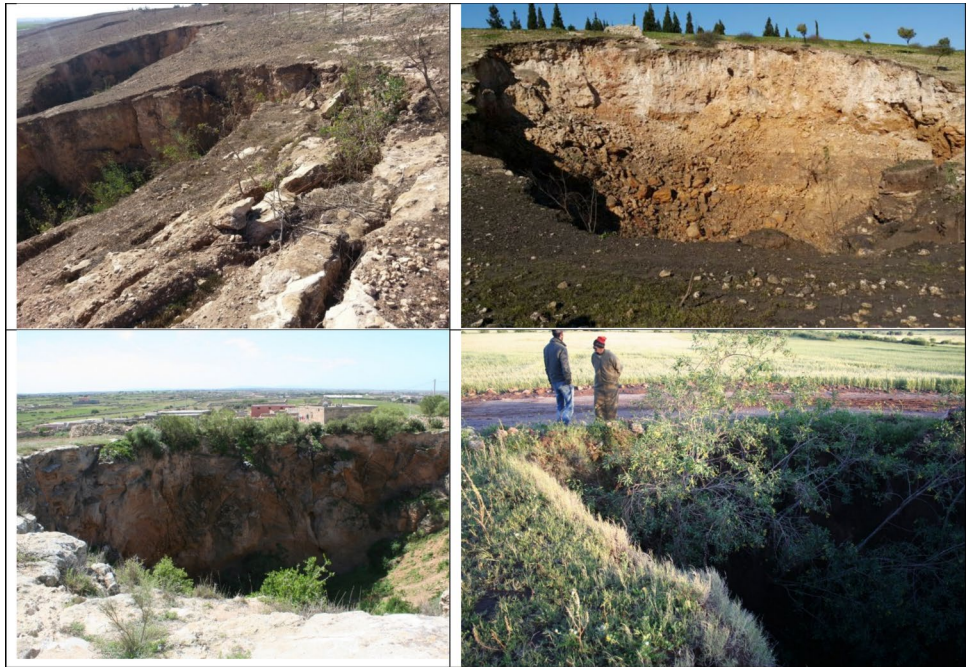
Fig. 4 Example of the sinkhole collapse in the study area
