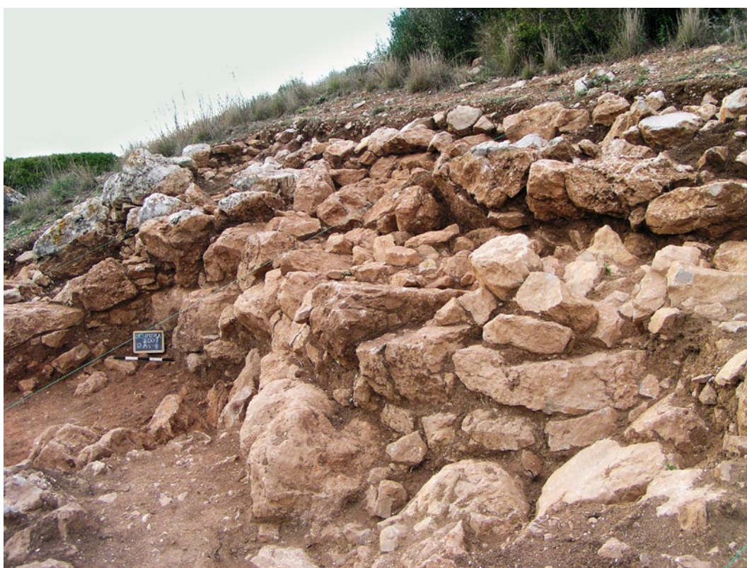
Fig. 8 Outeiro Redondo. Detail of the western side of Wall G, corresponding to the longitudinal overlap of several stretches, forming parapets along the steep slope.
